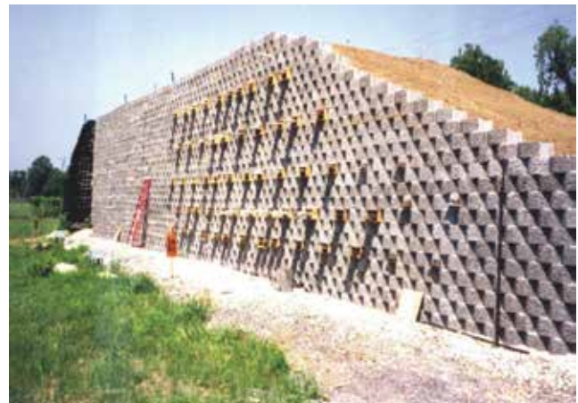
Figure 20. Reinforced soil retaining wall prepared for field reinforcement pullout test [58]
