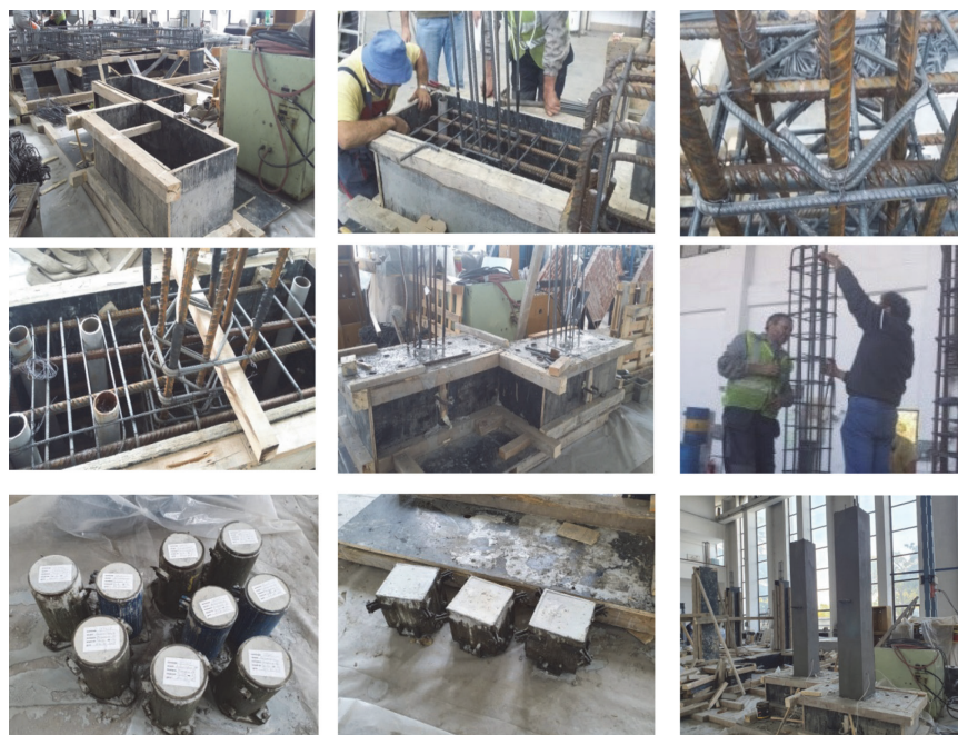
Figure 3. Construction of column models (Model M1 and Model M2) for experimental test
